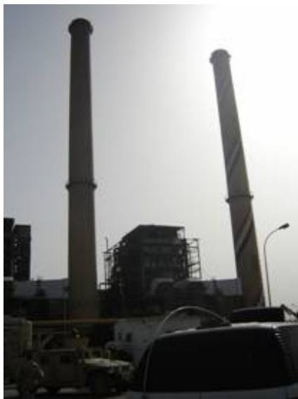
Photograph showing two of the four smokestacks at the Doura Power Plant which will remain dormant until the two turbine generators for units 5 and 6 are put back into operation. (Baghdad, Iraq; March 2005)
