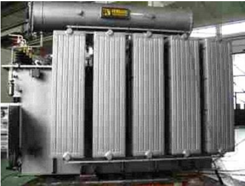
Photograph of one of the new transformers that Bechtel will be installing in each of the distribution substations that are being refurbished and constructed in the Baghdad area under one of the Mission's infrastructure projects. (Furnished by USAID/Iraq Mission; Baghdad, Iraq; February 2005)
