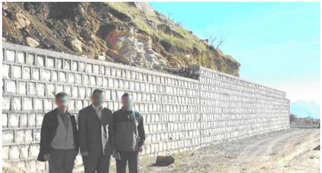
Photograph of one of a series of retaining walls constructed under USAID/Iraq’s Community Action Program in the town of Chwarta, Iraq. Photograph includes local government officials and an ACDI/VOCA 3 project engineer. Faces smudged for security reasons. (December 2004)
