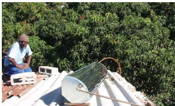
A local official in the Durban area of South Africa found low cost solar water heating simple enough that he installed it on his own.
