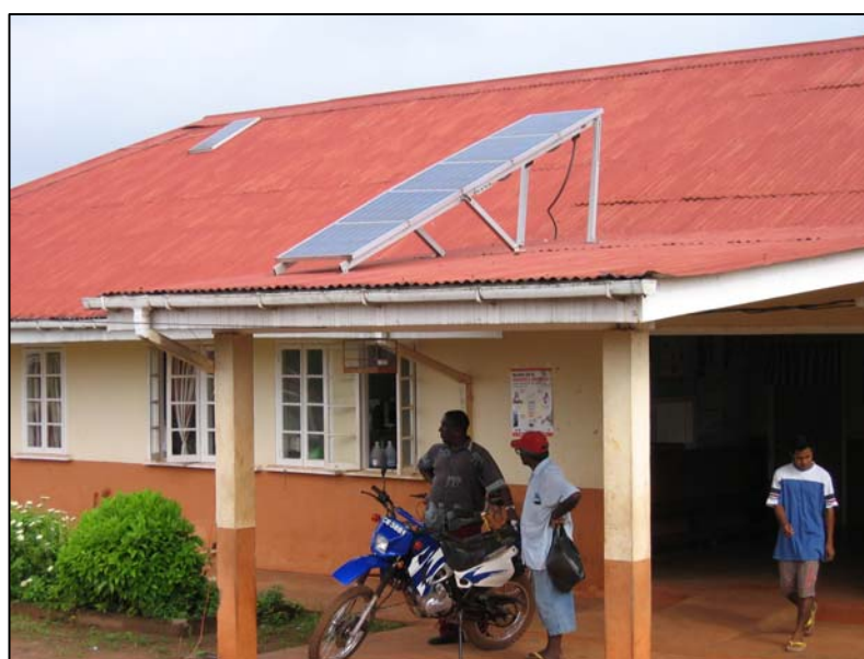
Unreliable supply of electricity is the #1 problem at the Mahdia Regional Hospital in Guyana.
