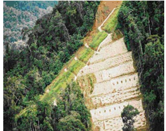
Section of ROW with revegetation and side slope with geotech mats
