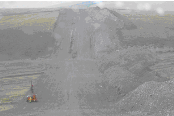
Pipeline right of way between the Qtsia Tabatskuri Protected Area (IUCN category IV) and Lake Tabatskuri. Unprotected topsoil lies to the right.
