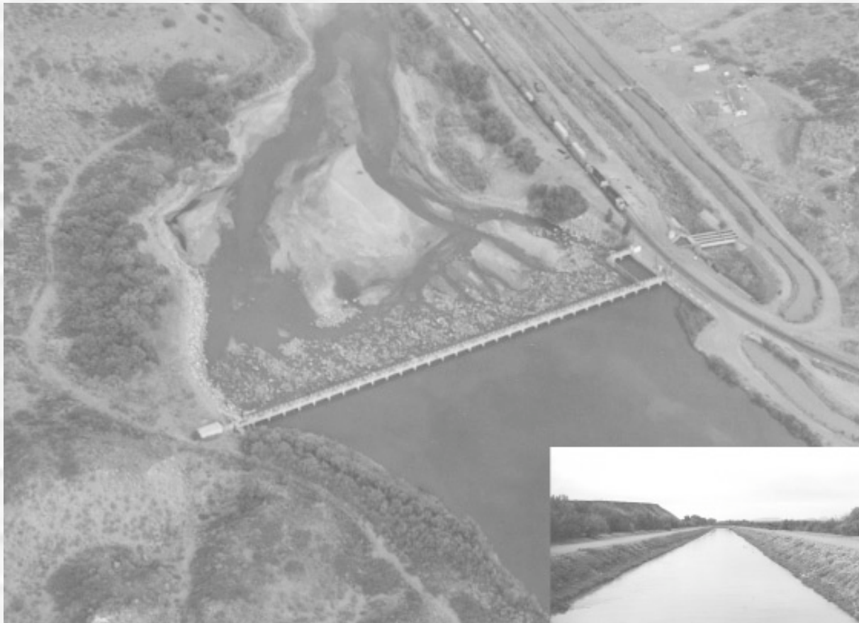
Figure 8 a & b. San Acacia Diversion Dam and Low Flow Conveyance Channel (inset), Socorro, New Mexico. (Photo courtesy of U.S. Fish & Wildlife Service)
