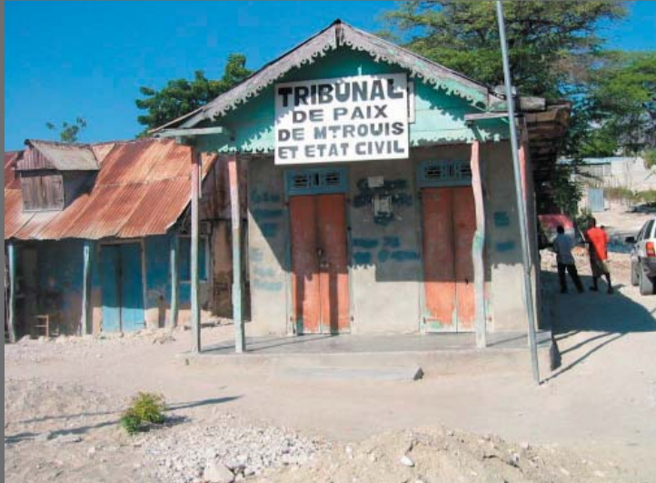
Photograph of Justice of the Peace Court House Montrouis, St-Marc, Haiti. This one-room courthouse had no running water or electricity.
