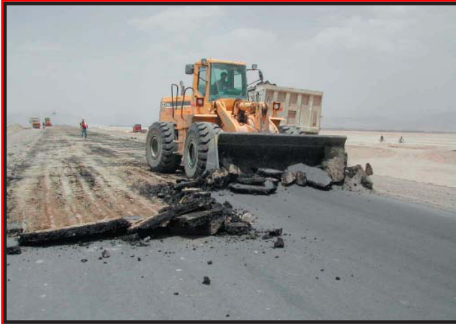
Photograph of a subcontractor removing defective asphalt. An OIG auditor and U.S. military personnel observing a subcontractor applying asphalt. The photographs were taken about 120 kilometers west of Kabul, Afghanistan.
