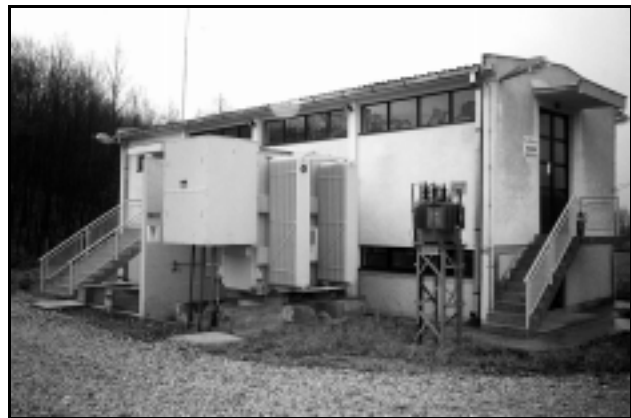
Figure 5 The new Kalesija substation.
