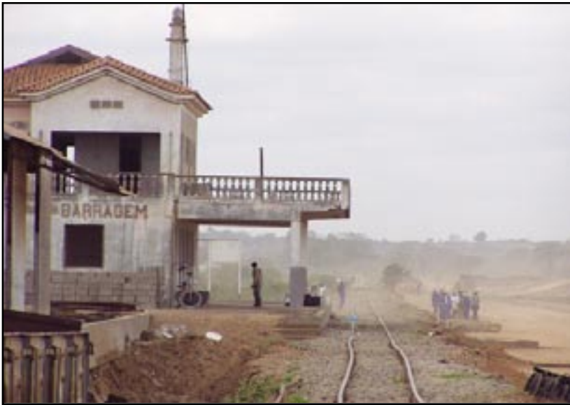
Photograph of railroad tracks and station near Macarretane, Mozambique. Floods waters in 2000 reached as high as the balcony overhanging the tracks.
