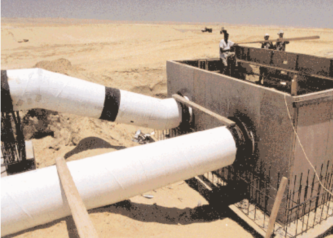
Construction of a portion of the wastewater project.
