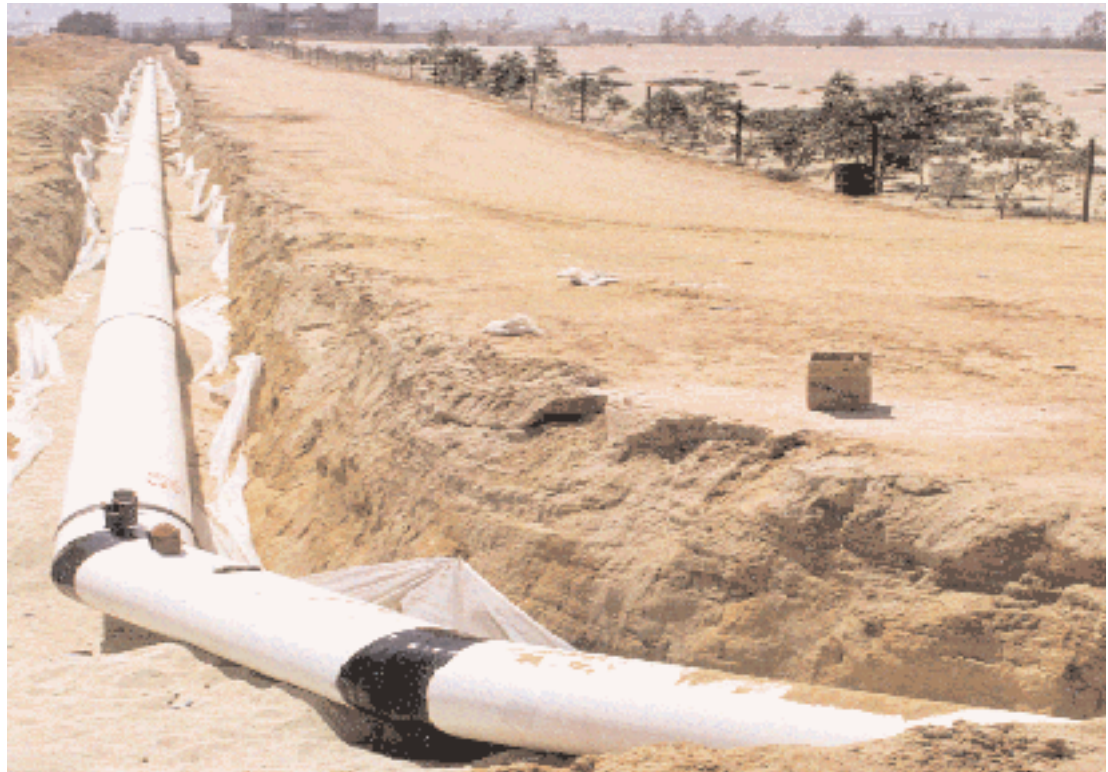
Piping being laid for wastewater treatment plant.
