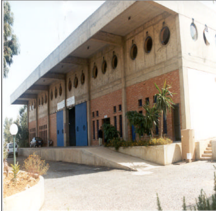
Moroccan Ministry of Health's USAID-funded warehouse built in Sale' for storing family planning commodities
