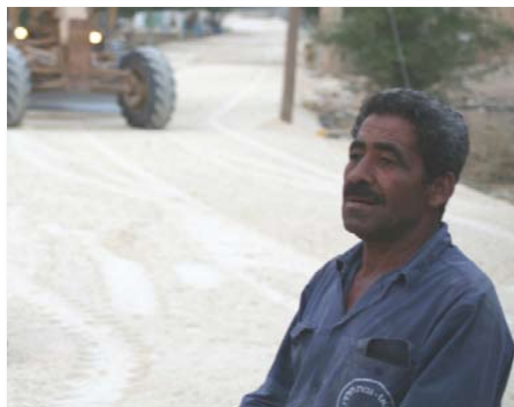
Farm worker Khalil Jalaith, 50, watched road construction near his home. He said that moving his disabled, 14-year-old son to treatment will become smoother and easier once the road is paved under the USAID-funded project.
