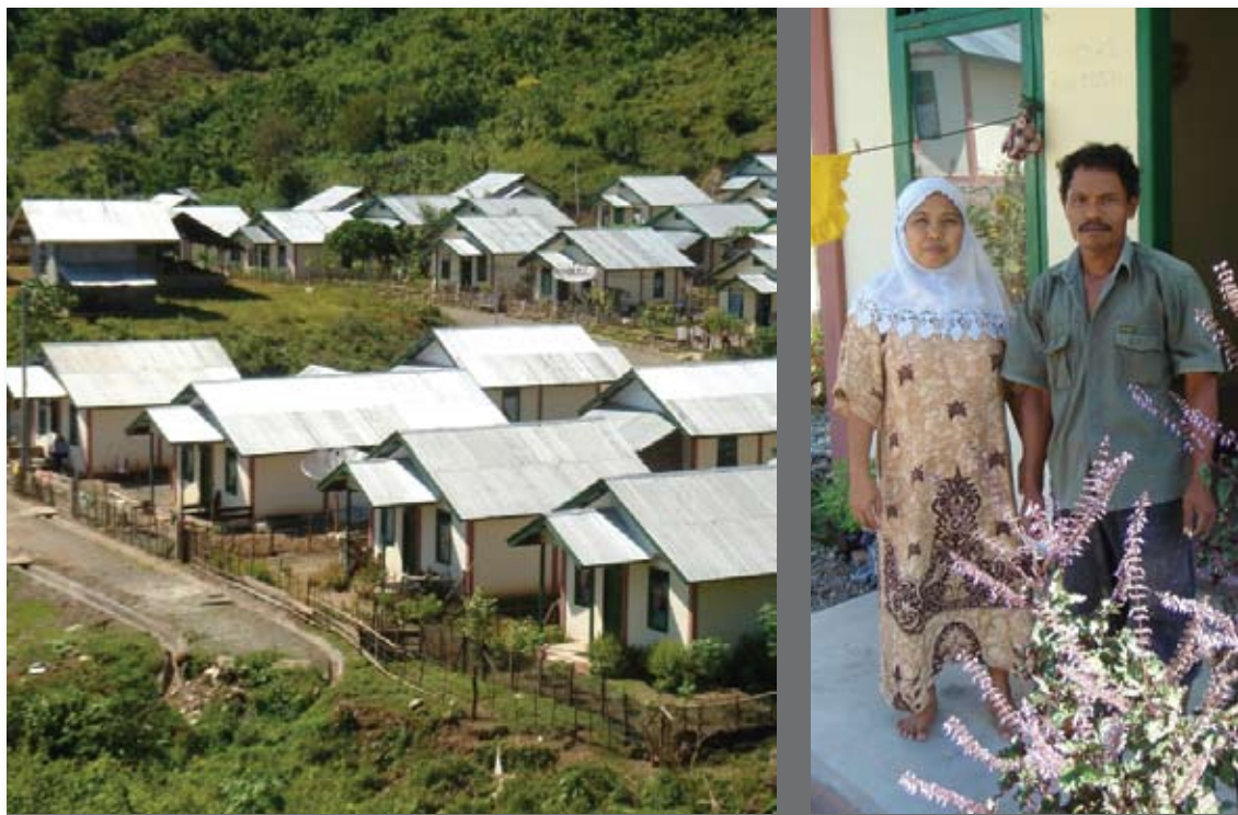
With an emphasis on quality and timely completion, USAID has funded the reconstruction of houses and roads in the village of Babah le, Banda Aceh, Indonesia. Residents pose in front of their newly constructed home.
