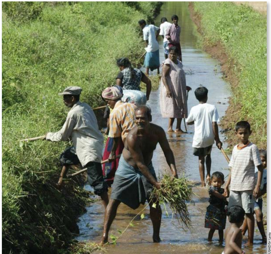
Sinhalese and Tamil communities in the Trincomalee District in Sri Lanka—overcoming tensions fostered by extremists on both sides—come together to clear debris from a tsunami-damaged canal under a USAID-funded infrastructure grant.
