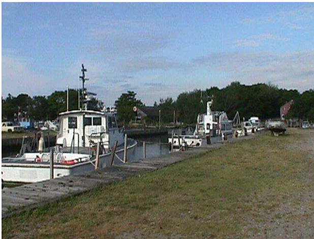
Figure 1-7. Fire Island National Seashore marina
