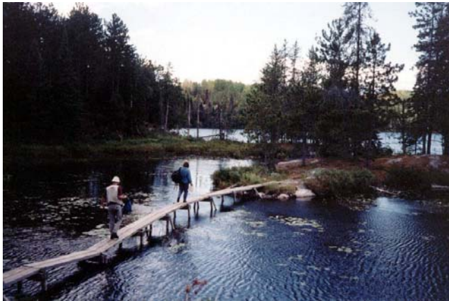
Figure 11-18. Boardwalk at Cruiser Lake picnic site
