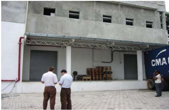
Photo of the Partnership's new central warehouse taken by an OIG auditor in Port-au-Prince, on May 29, 2008.
