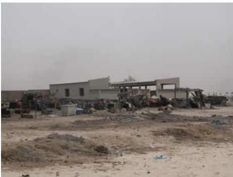
Newly constructed building at the fish-processing site of Bok Khalaat. According to the 1-year grant agreement, ADF was to provide funding for site improvements for the women processing fish on the beachfront. Photograph taken by an OIG auditor on January 17, 2008.
