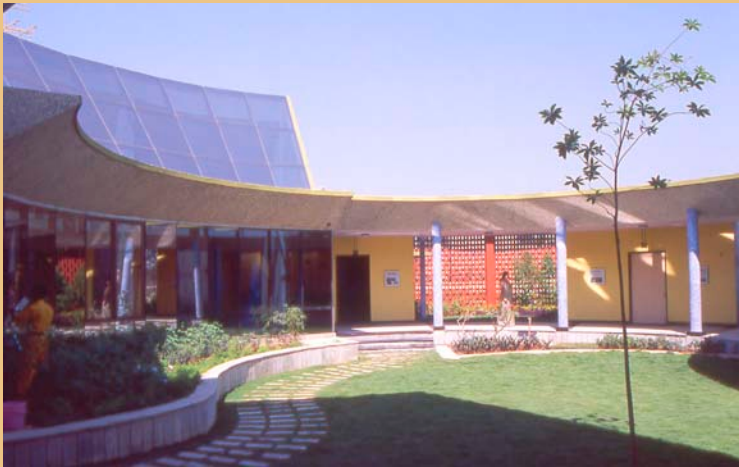
The Green Business Center in Hyderabad, India.
