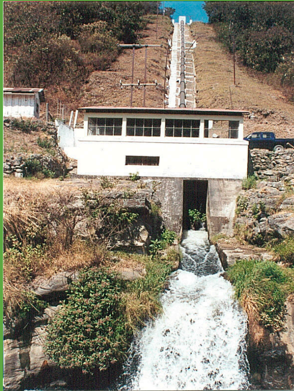
La Castalia, municipal hydroelectric plant in San Marcos, Guatemala, is supported by the FENERCA program.
