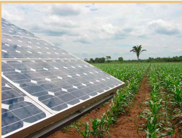
Village Energia Ambiental photovoltaic powered irrigation system, Brazil.
