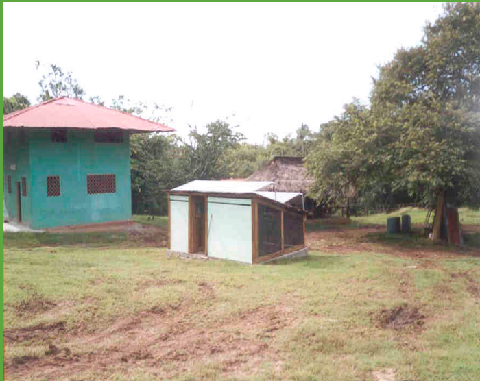
Center for Environmental Studies with a photovoltaic system – ANCON- National Park Punta Patiño, Panama.
