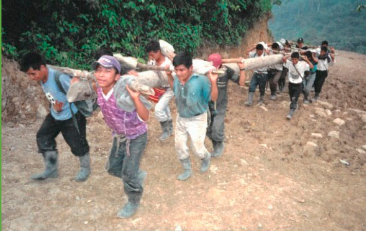
Local workers carrying construction materials for the micro-hydroelectric plant.
