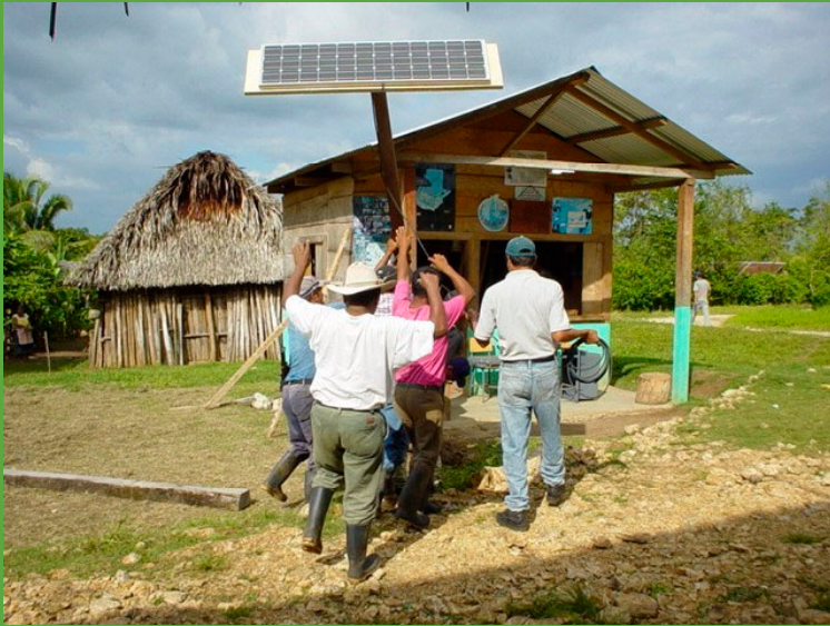
Installing photovoltaics for communications and lighting in Cancuén National Park.
