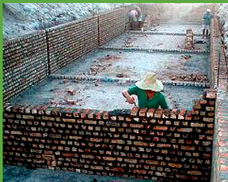
Cabocharde community constructing the reservoir.
