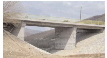
The Orlan Bridge in Podujevo Municipality was restored by USAID / CISP
