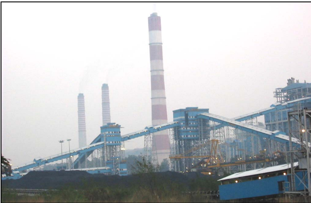
Office of Inspector General photograph of the Vindhyachal Super Thermal Power Station in Madhya Pradesh, India, where greenhouse gas project activities were implemented (February 2008).
