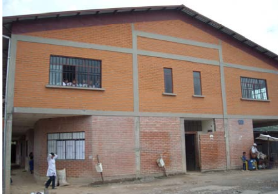
An estimated 570 students from Huancané and the surrounding communities attend primary and middle school in this building. Photo taken by a RIG/San Salvador auditor on April 9, 2008.
