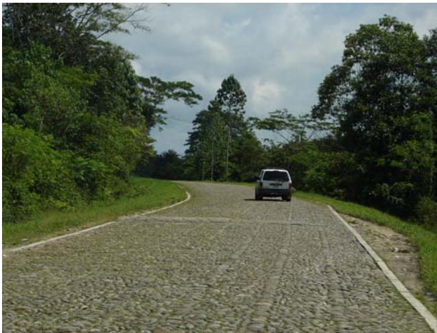
A road in the Chapare region supported by the USAID/Bolivia's Rural Roads Authority Project. Photo taken by a RIG auditor on April 10, 2008.
