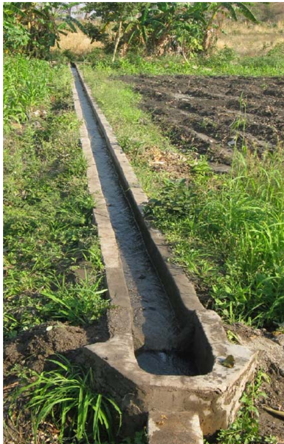
A feeder channel built through the RIPE program diverts water from the Mpmemba stream and irrigates farmers' fields (Photo by Alexandra Riboul, USAID).
