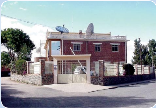
USAID's former office building in Asmara, Eritrea with inadequate setback from street. PHOTO: USAID/OFFICE OF SECURITY (SEC)
