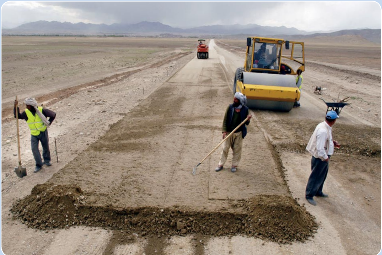
Workers build a road from Ghazni to Gardez, linking the region to the main highway connecting Kabul to major cities.
