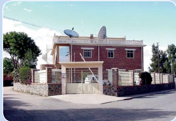
USAID's former office building in Asmara, Eritrea with inadequate setback from street. PHOTO: USAID/OFFICE OF SECURITY (SEC)
