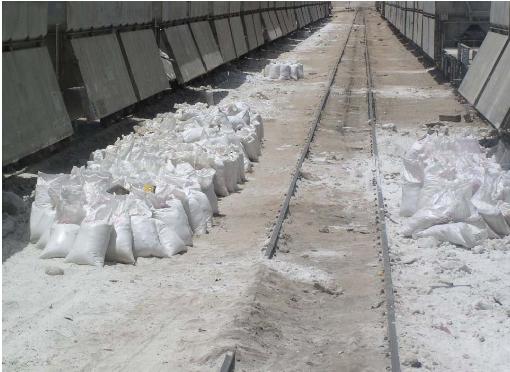
Figure 2. Main line north of Umm Qasr with evidence of looting of bulk ammonia.
