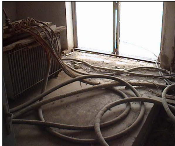
Figure 19 In addition to the panels, general cable runs need attention. Here, a 415 V, three-phase supply from the generator has been pulled into the transformer room with little concern for hazards around the draw pit.
