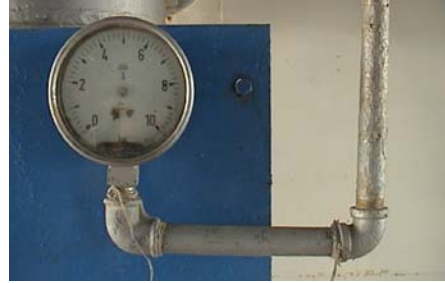
Figure 7 Many gauges will require replacement; all will require functionality checks.
