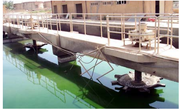
Idle Ad Diwaniyah Water Treatment Plant
