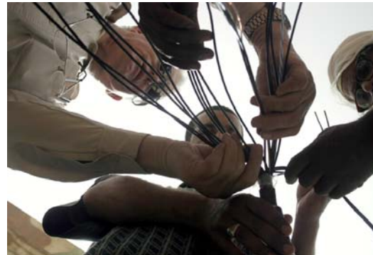
Dilapidated port wiring
