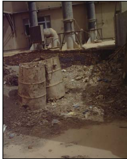
Figure 28 Often, only a general cleanup is required.
