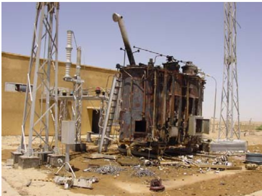
Burned Transformer
