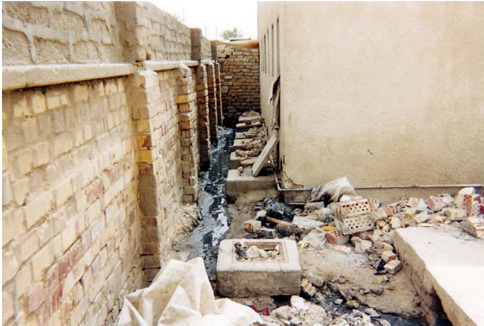
Debris and Building Waste in School Yard
