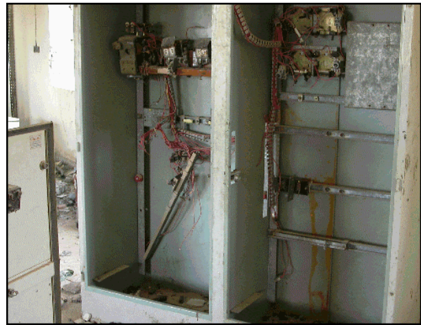
Figure 13 Copper content within the enclosures has been removed.
