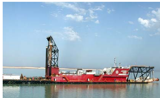
Dredging Equipment – Umm Qasr Port
