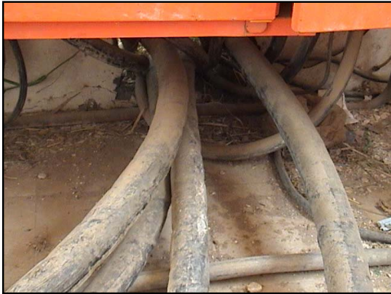
Figure 10 Holes and gaps in cables need to be filled using foam.
