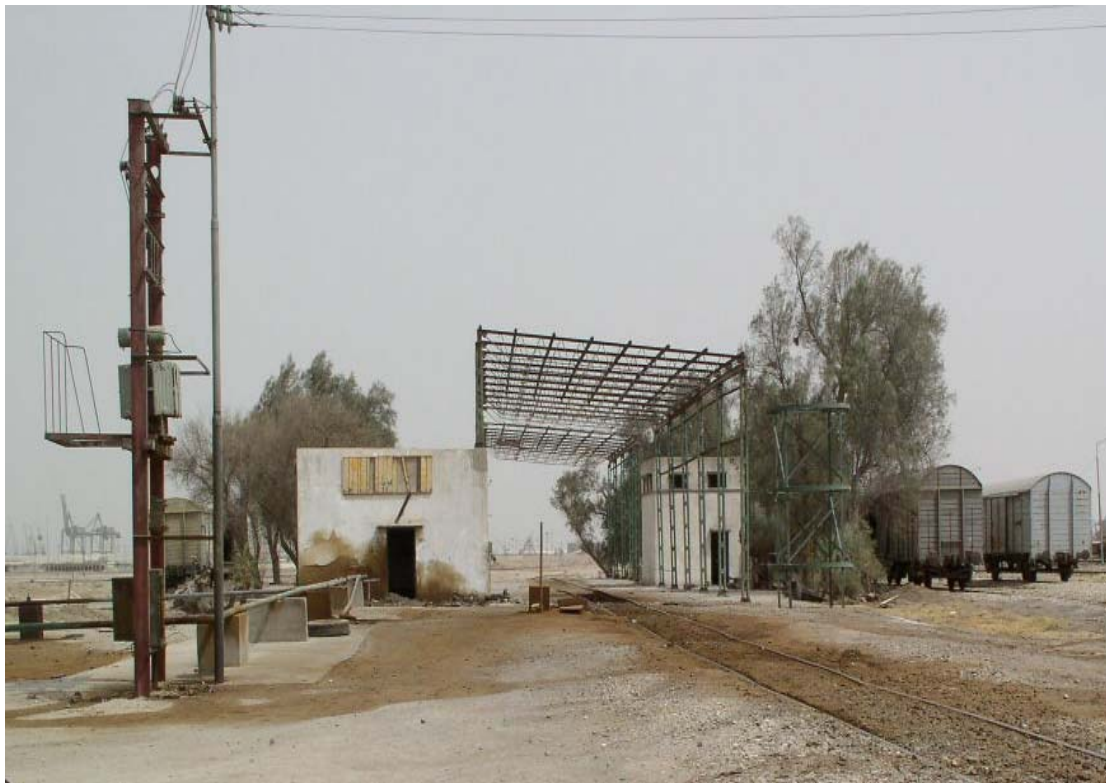
Figure 6. Umm Qasr shed with stolen roof, water tank, and fuelling equipment. Note also heavy ground pollution.
