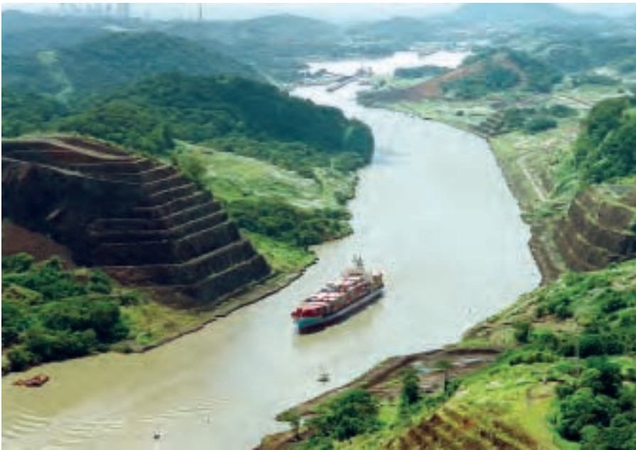
PANAMA CANAL: The flow of the Panama canal, which carries 40 percent of U.S. international trade, depends on an abundant supply of fresh water from surrounding hills. USAID works to preserve protected areas that harbor high biodiversity and also provide a steady stream of fresh water.
