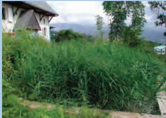
ARTIFICIAL WETLAND (before and after): The Pisgah elementary school treats its septic wastes using this wetland created with rocks and local reed grasses, producing virtually pure water for release into the watershed.
