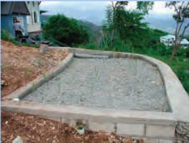
ARTIFICIAL WETLAND (before and after): The Pisgah elementary school treats its septic wastes using this wetland created with rocks and local reed grasses, producing virtually pure water for release into the watershed.
