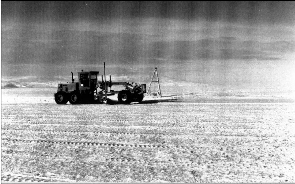
Figure 2. Laser-controlled grader used to level natural ice surface for runway.
