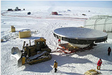
Transporting the 10-meter dish to be installed on the pedestal at Amundsen-Scott South Pole Station. This new telescope will gather information on cosmic microwave background radiation. (NSF/USAP photo by Bill Johnson)
