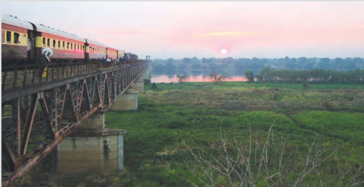
Sunrise at the restored Zofu Bridge greets train passengers in eastern DRC.
