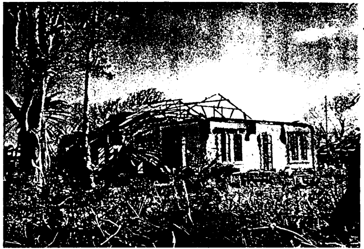
A house in Farafangana destroyed by the force of Cyclone Gretelle.
