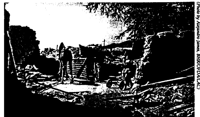
Rubble of homes in Nazca, Ica Province.
