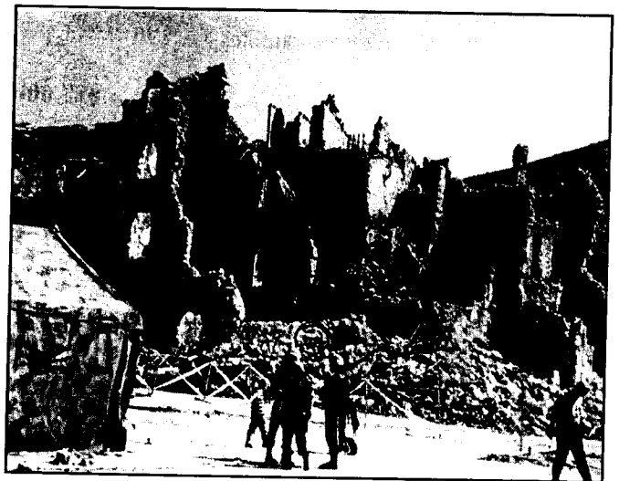
The front line in Mostar, Bosnia-Herzegovina.
