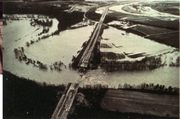
The New York State Thruway bridge over Schoharie Creek near Amsterdam, New York, collapsed on April 5, 1987, claiming 10 lives, after the foundation soils under a pier footing were washed away during a severe flood. (Photograph by Sid Brown, Schenectady Gazette, used by permission)
