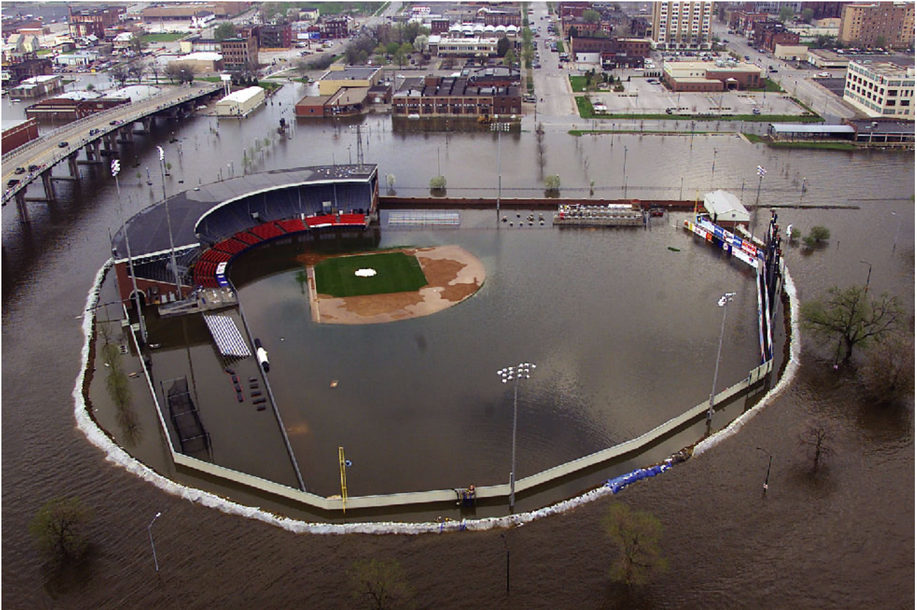
Melting snow and heavy spring rain combined to cause severe flooding on the upper Mississippi River in April 2001. Davenport, Iowa, was particularly hard-hit. In this photograph, all but the infield of John O'Donnell Stadium, home of the Quad Cities River Bandits, lies underwater. The record Mississippi River flood of 1993, caused by a persistent mesoscale convective complex, along with other cities in the Mississippi Basin. (Photograph by John Schultz, Quad Cities Times, used by permission.)
