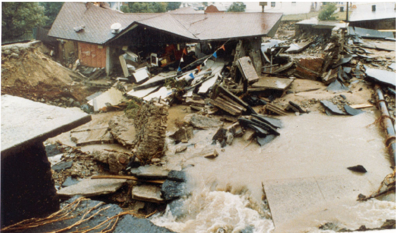
Persistent, widespread torrential rainfall caused flooding across central Michigan in September 1986, resulting in unprecedented damage. (Photograph by Scott Harnesen, Bay City Times, used by permission.)
