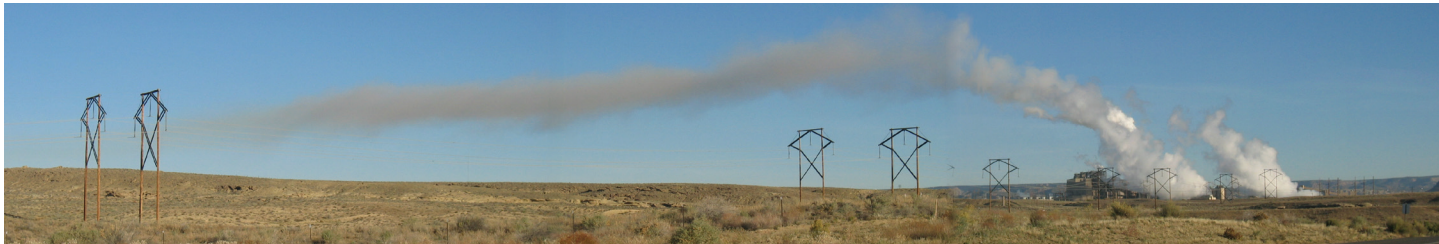
Figure 1. Typical emission plume from a powerplant near Shiprock, New Mexico, is horizontal during an inversion October 26, 2003; inversions are more common in winter than summer. Photograph copyright (2003) Diane J. Schmidt, all rights reserved; used with permission.
