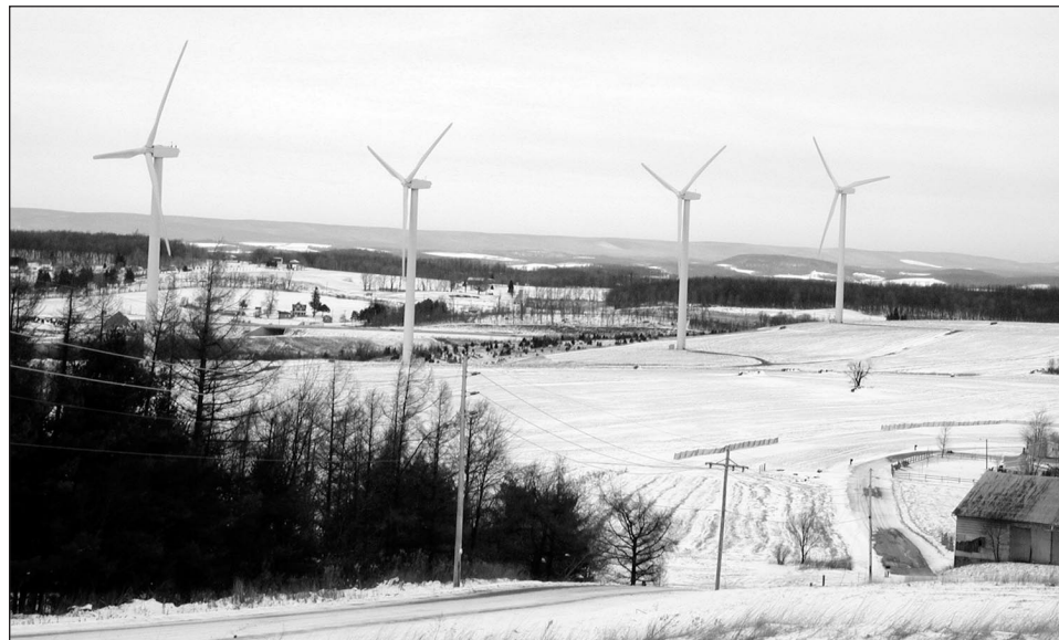
Figure 6: Wind Power Facility in Somerset County, Pennsylvania
