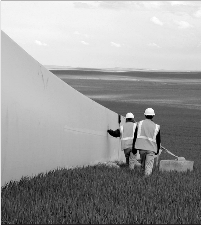
Figure 5: Wind Power Facility in Sherman County, Oregon
