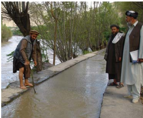
WATER CONTROL: Officials check the water flow in a 400-year-old canal along a major river in Badakshan Province, repaired through international assistance so farmers can irrigate crops.
