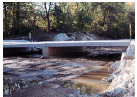
Newly completed open-span low water crossing over Thomas Creek will allow Niangua darters and other aquatic species to pass freely.
