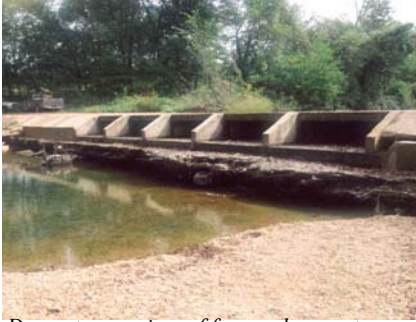
Downstream view of former low-water crossing over Thomas Creek.
