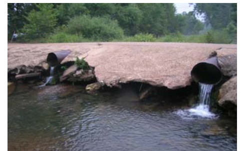
Example of crossing with perched culverts in Missouri Ozarks
