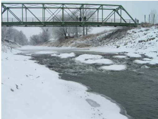
Newly created riffle approach to Seven Mile Creek weir.
