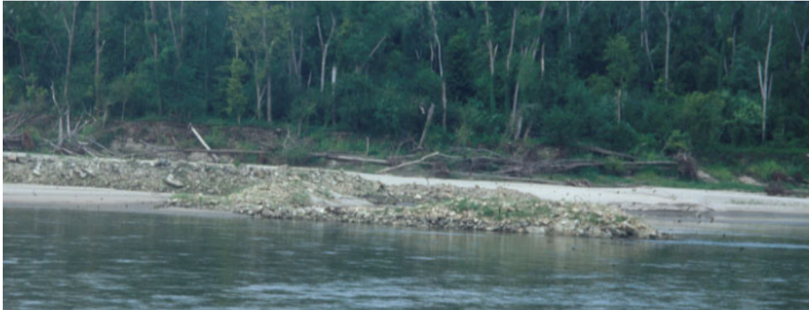
Typical wing-dike habitat with a scour hole downstream associated with a sand bar
