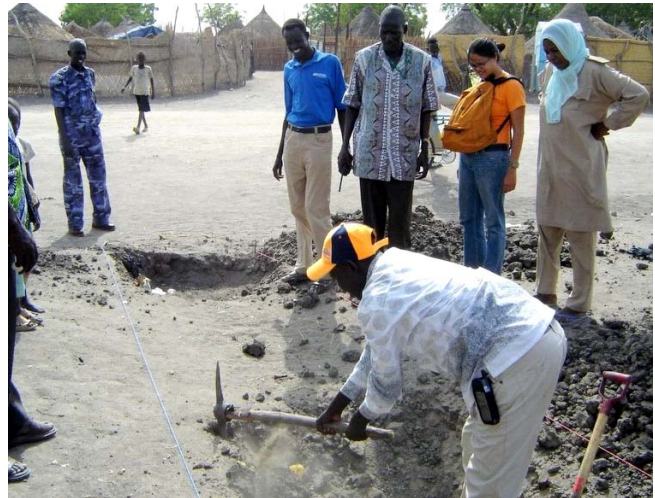
Local laborers improve basic services in Malakal, Upper Nile. Photo: USAID
