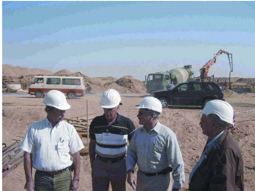
Critical human resources are also needed to address strategic priorities such as those in the Middle East. In this photo, the USAID/Jordan Water Resources Office Director James Franckiewicz reviews the progress of work at the Aqaba Wastewater Treatment Plant.
