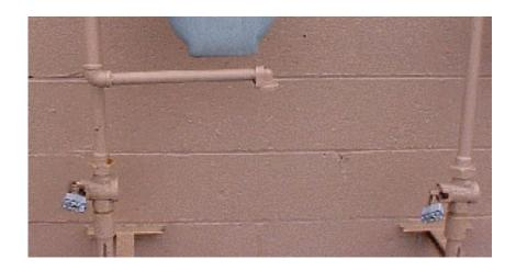
• <u>Riser misuse</u>. The tenants or customers should not be permitted to use the riser and its components for other purposes. Never use the riser as an anchor for laundry lines, plant supports or bicycle racks.
