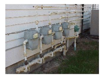
A good coating of light colored metallic paint on all aboveground piping subject to corrosion provides sufficient protection to retard corrosion. The point where the riser comes out of the ground is susceptible to corrosion on metallic risers and should be inspected periodically.
