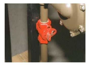
Valves used with polyethylene pipe and tubing must meet the requirements of ASTM D2513 and be so marked.
