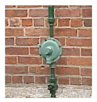
It must be remembered that this means of accomplishing overpressure protection operates by releasing propane to the atmosphere instead of inside a building in the event of a failure. Operators of small propane systems may elect to advise their customers of the need to report any releases of propane which will be identified by an obvious hissing noise coming from either regulator.
