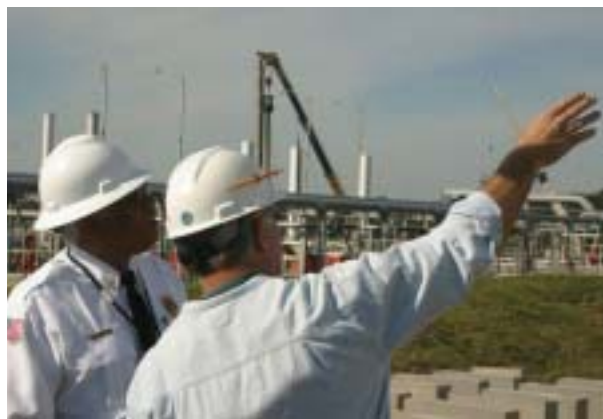
Figure 1 A State Fire Marshal inspects an LNG tank under construction.
