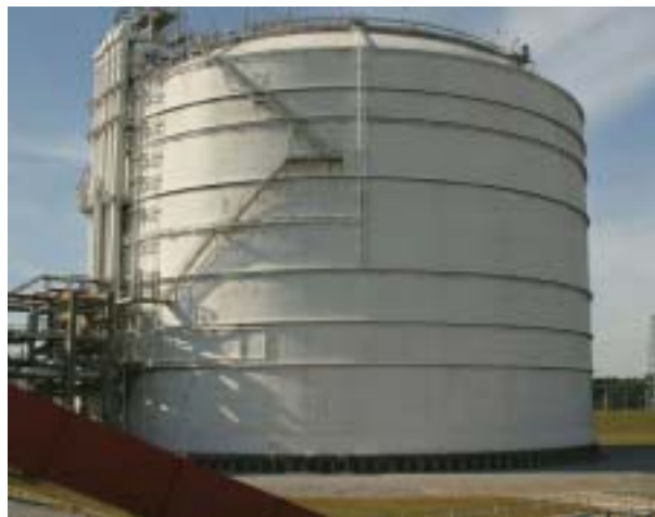
Figure 5 LNG tanks are surrounded by impoundment areas capable of containing 110% of the maximum storage capacity.
