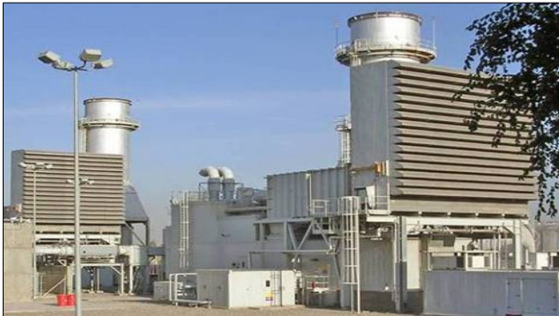
Newly constructed Baghdad South: Units 1A and 1B
