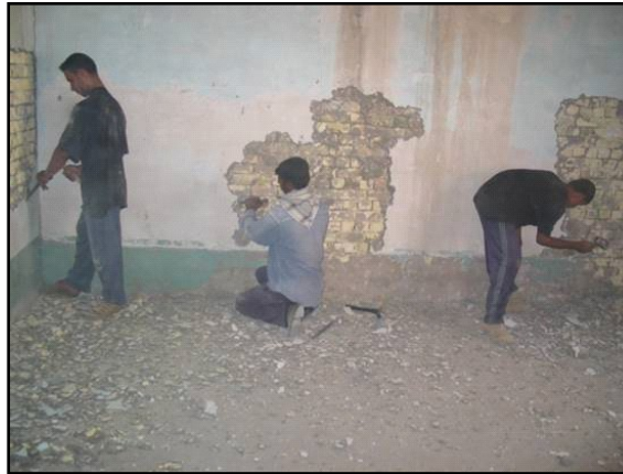
Library reconstruction project in Maysan Governorate
