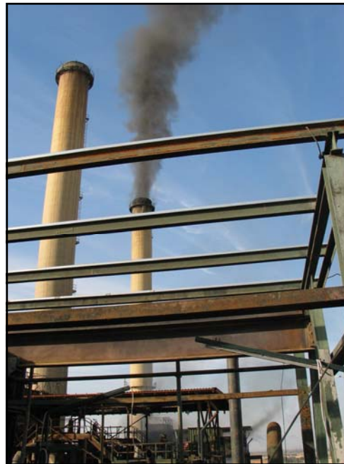
A USAID power plant restoration project
