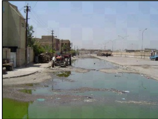
Contaminated water leaking into Baghdad neighborhood streets
