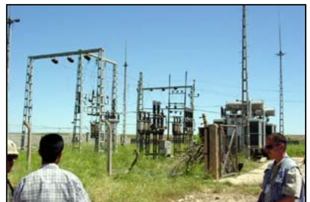
Bechtel assessment team inspects power infrastructure in northern Iraq. (Photo: Bechtel National, Inc.)
